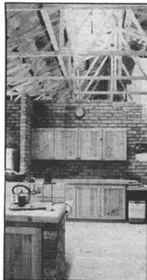
The central area in the solar home is this large country kitchen. Large amounts of brickwork increase the home's thermal mass so that it retains heat more in the winter, while the open space between the walls and ceiling allows a free flow of air though the house.
