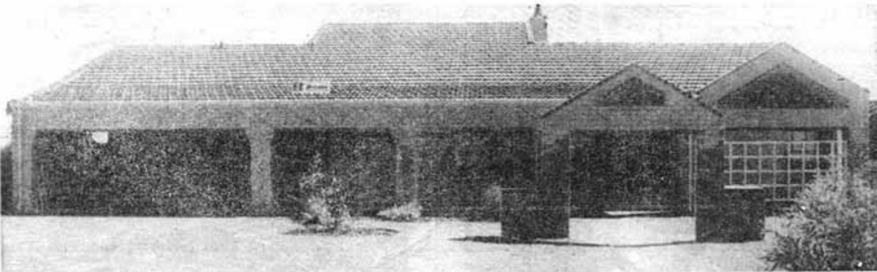
The front veranda of the solar energy ideas display home at Kardinya keeps the early morning and late afternoon sun off the facade but, more importantly, keeps the ground cool in front of the bedroom windows.
