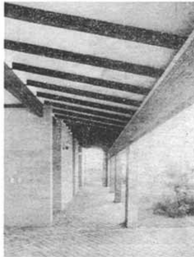
BELOW: The front veranda channels cooling air to the bedrooms in summer.
