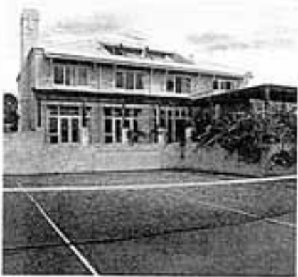
Facing page inset: Thick limestone is perfect high thermal mass material.
