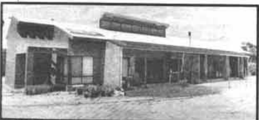
THE solar house windows face north and a pergola is designed to let in the winter sun and block the hot summer rays
