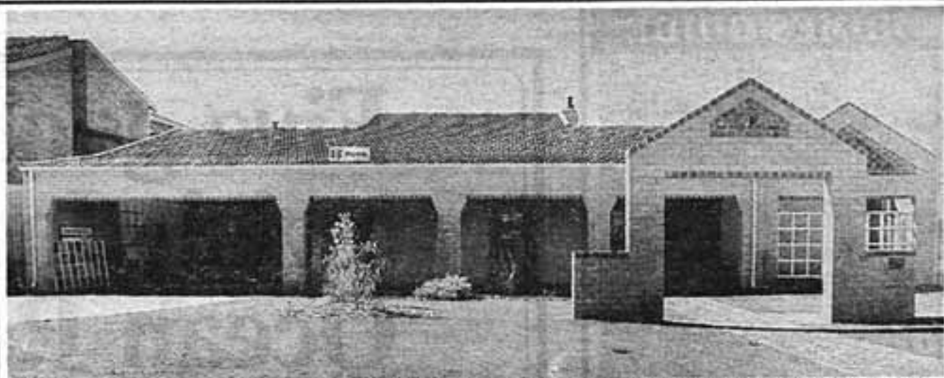
□ The recessed windows and choice of light-colored bricks are just some of the energy-saving ideas in this Bristle-Whittakers Solar Energy display home.
