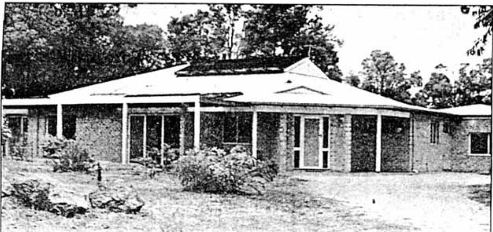
This passive solar home has been designed to harmonise with its environment.
