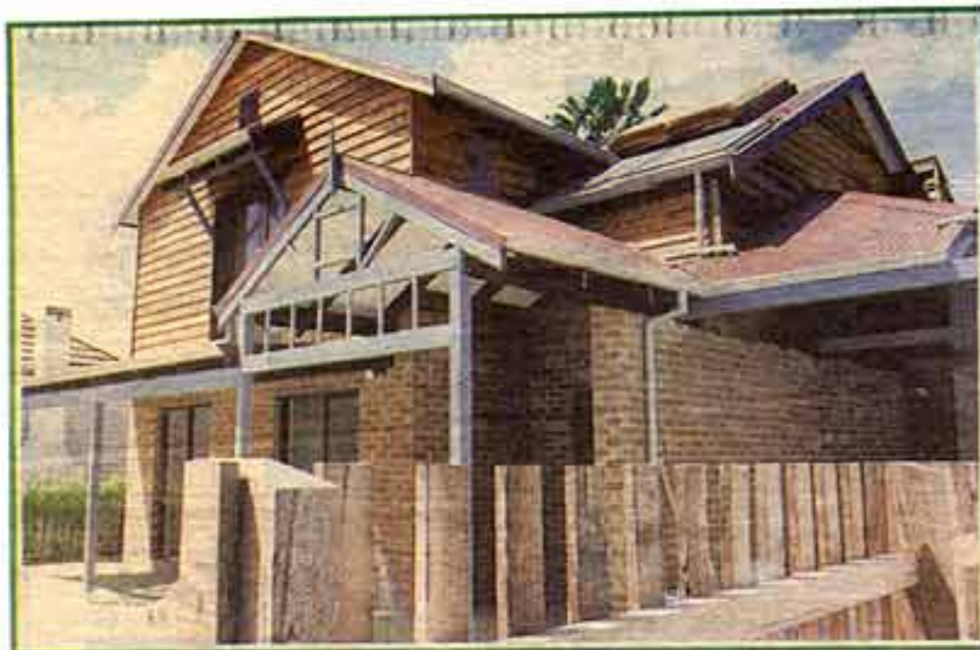
Western red cedar and brick make the house blend with its older neighbours.
