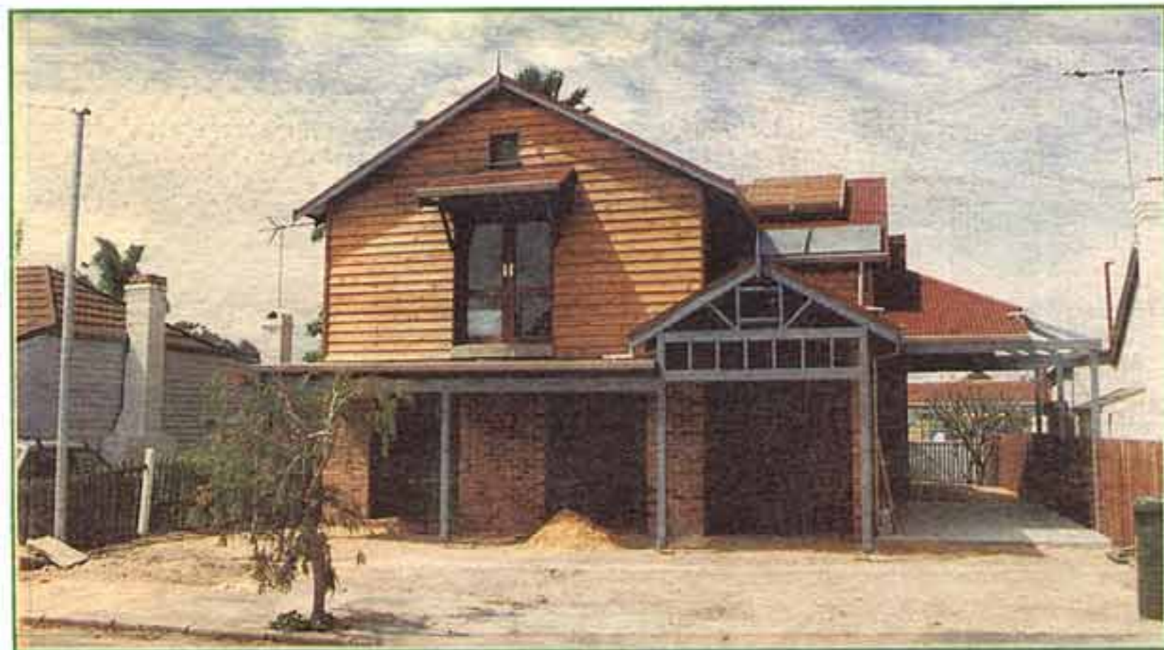
The front doors and windows on the ground floor are well screened from the sun.
