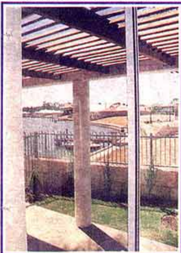
Sunlight is just starting to filter through solar pergolas as autumn begins.
