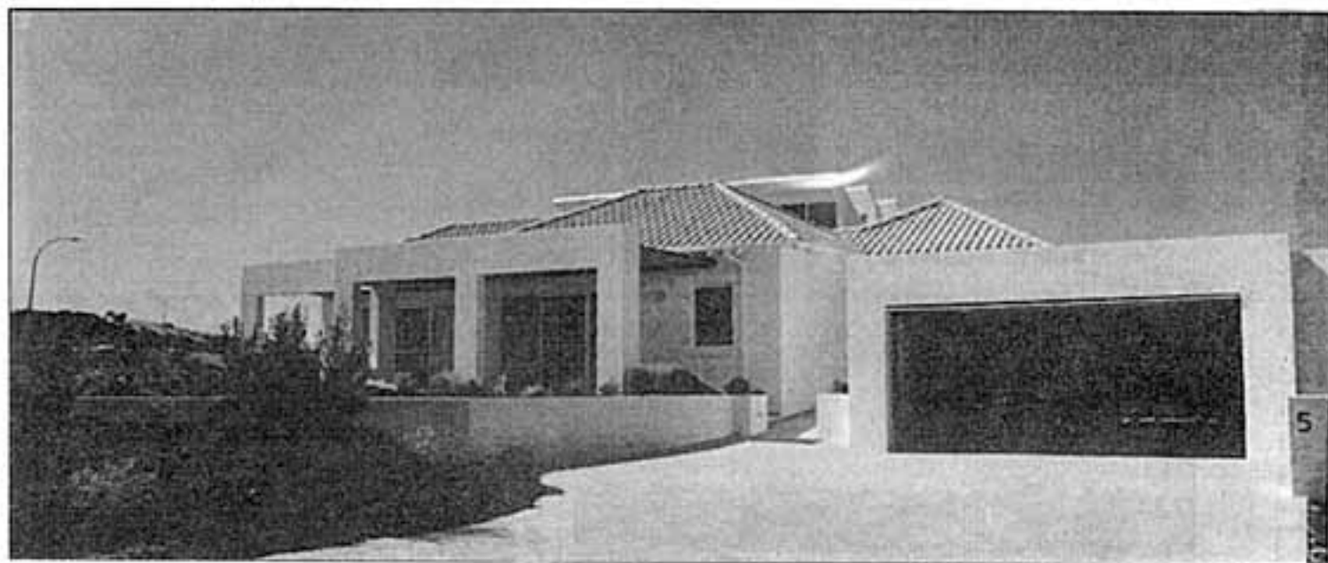
The passive solar house at Mindarie Keys makes the most of the Perth climate and the beach environment.
