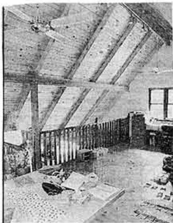
The studio loft has a sweeping, cathedral-like ceiling.
