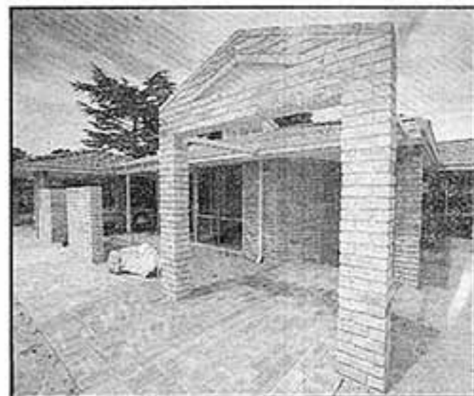
A brick gateway with gable top provides a dramatic entry.
