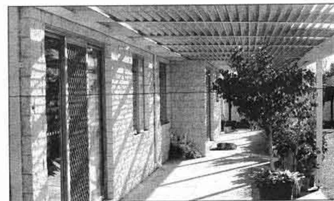
Louvres provide maximum sun during winter and shade in summer.
