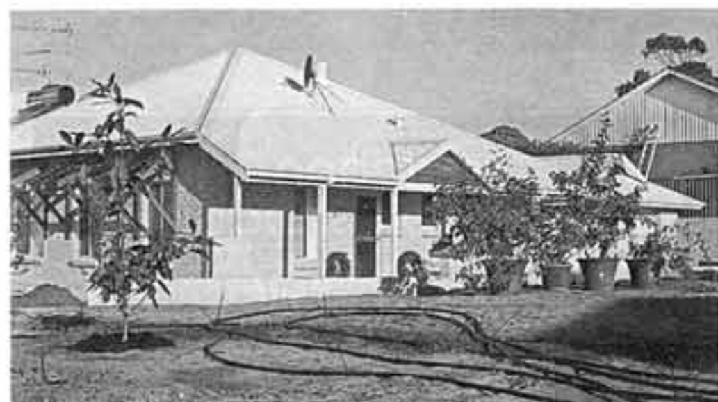
Verandas around the home are positioned to keep out the summer sun.
