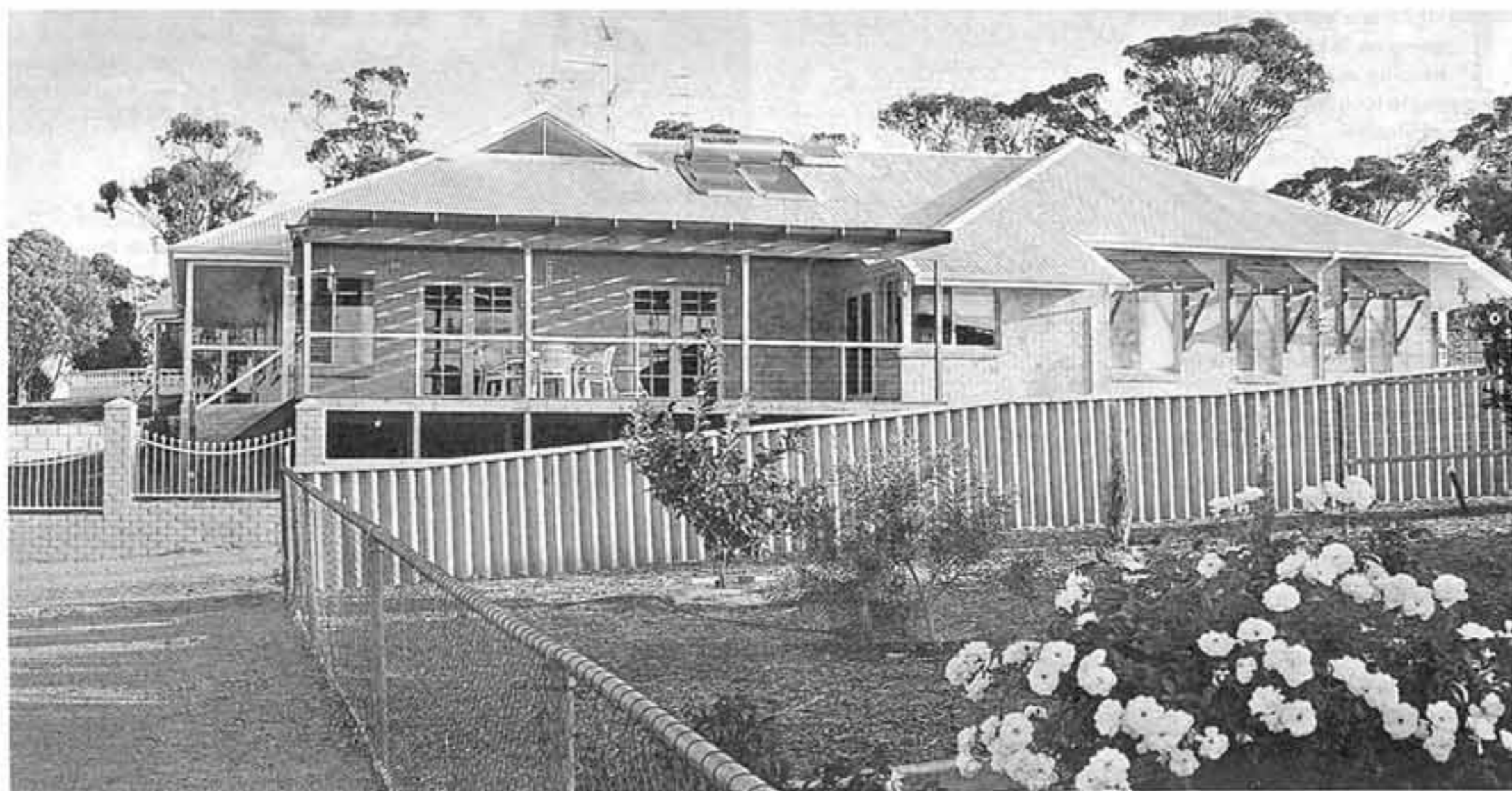
This homestead in the Wheatbelt town of Pingelly has been built using passive-solar principles.
