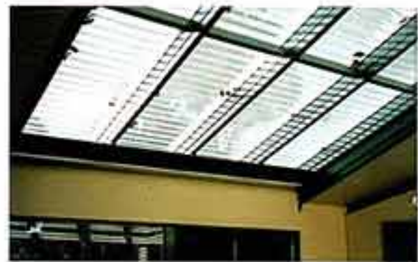
Below: Two detailed views of the Zoo building. First, looking up to the glazed internal atrium roof, showing solar control blades and second, the solar pergola, making the most of winter sunlight while keeping summer sun at bay.
