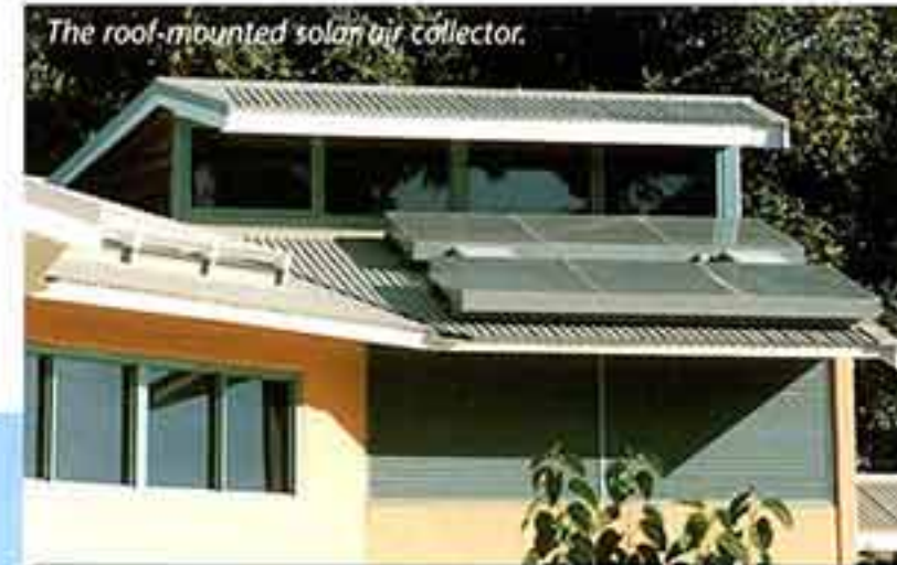
The roof-mounted solar air collector.
