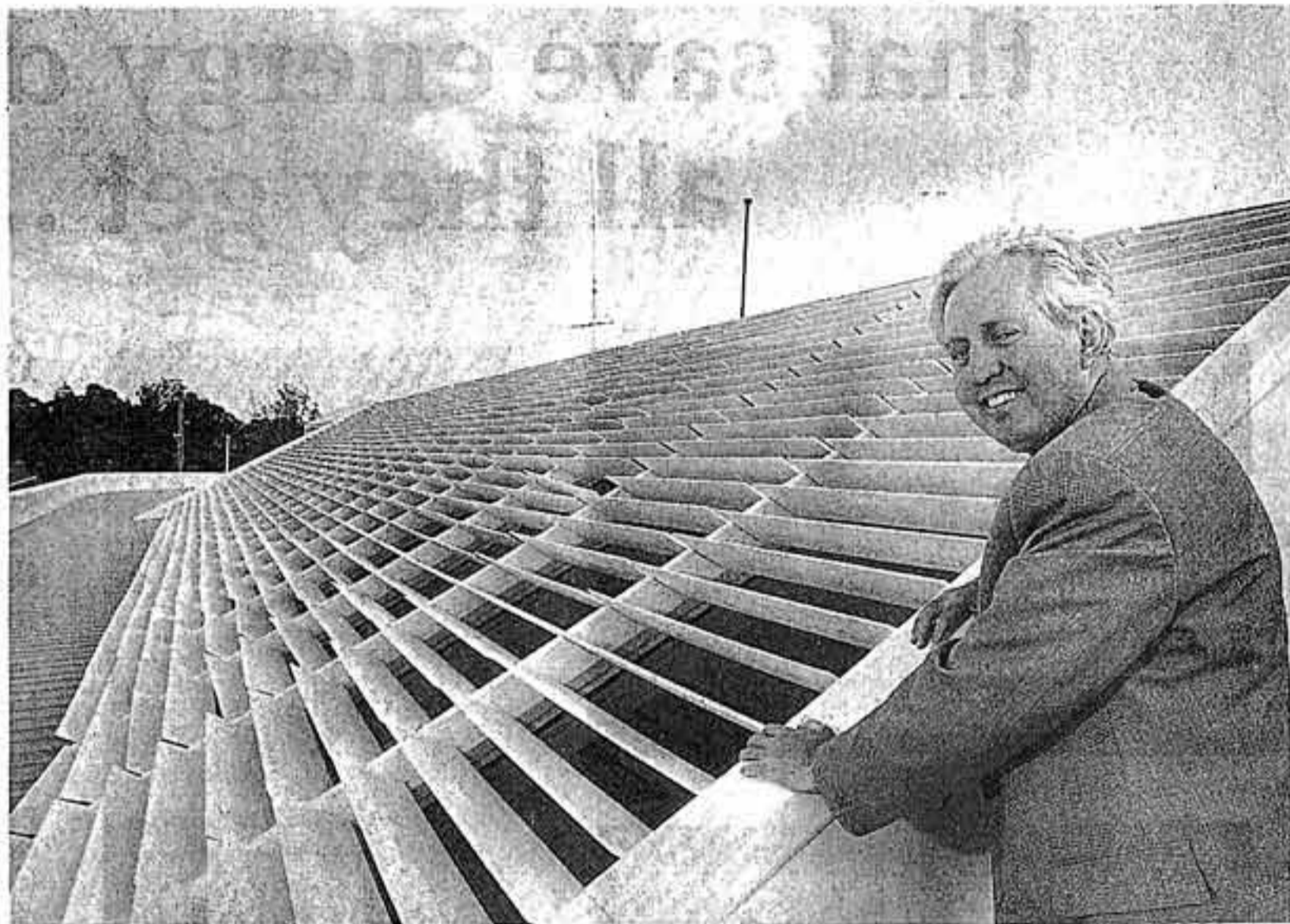
Let the sunshine in: Mr Baverstock demonstrates the louvre designed windows that allow in the light — Picture: Ken Matts
