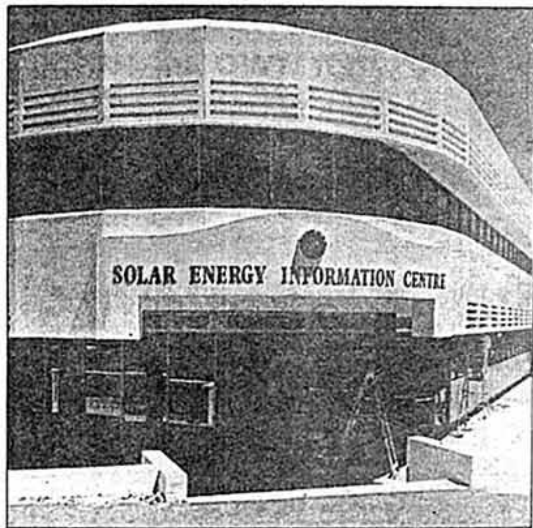
The new Solar Information Centre in Canning Highway, Como.
