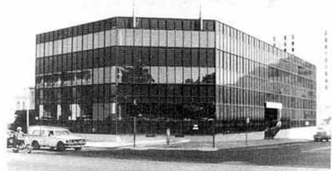
To refresh the memory of members, this photograph shows the building as it was when the League bought it in 1983. On the right of the picture can be seen the entrance in Bennett Street and the steps which had to be climbed.
