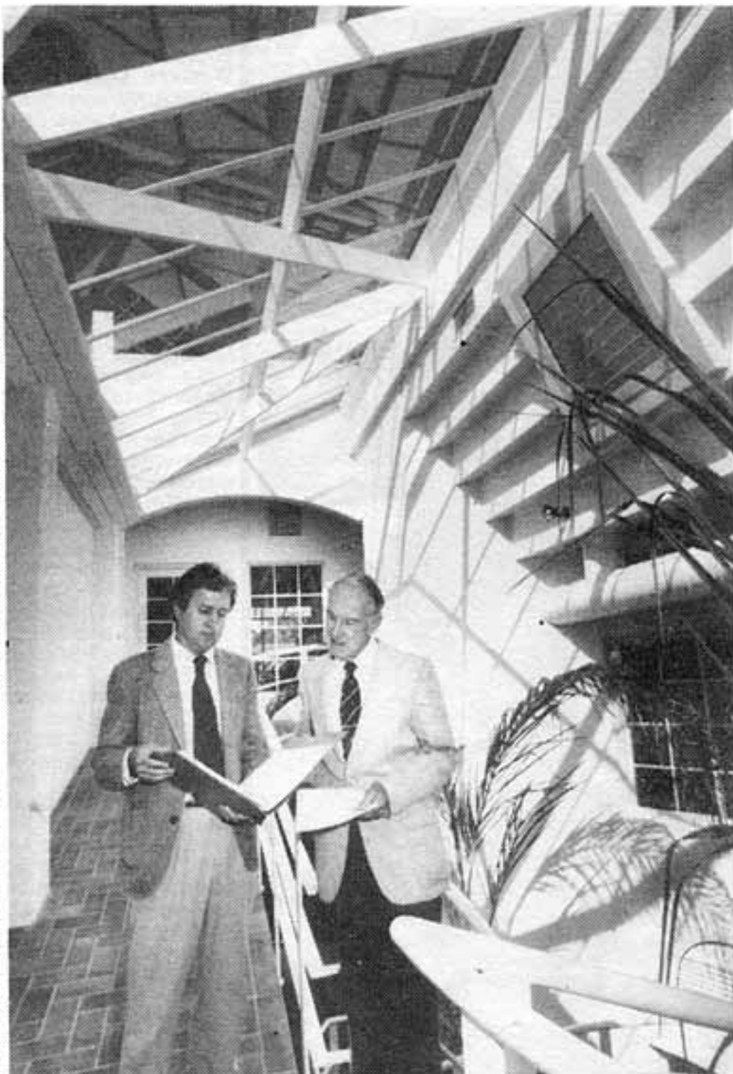
Solar Housing Interest Group secretary Rex Charles studies the design of a Gary Baverstock building in Subiaco, under the glass panels of the building. Air heated by the sun is ducted into the offices during winter.
