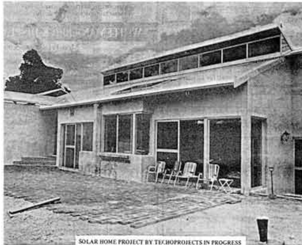
SOLAR HOME PROJECT BY TECHOPROJECTS IN PROGRESS
